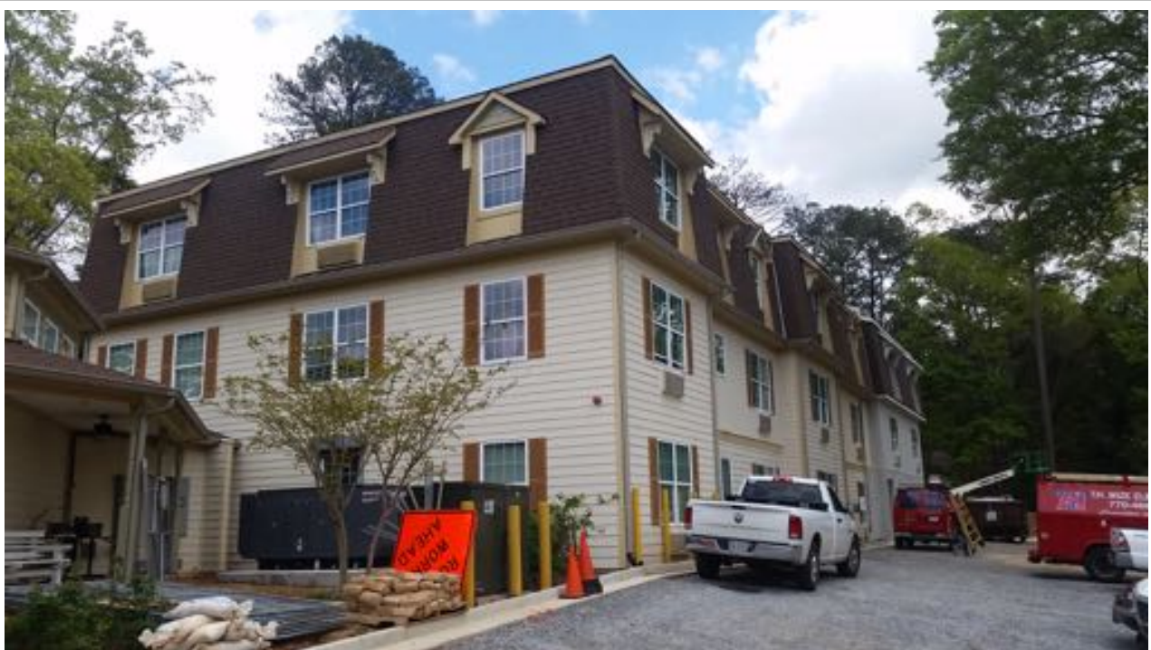
New Memory Care wing nearing completion at Peregrin's Landing in Atlanta.
